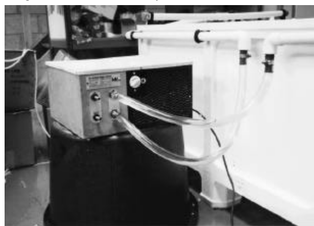
In-line seawater chiller
