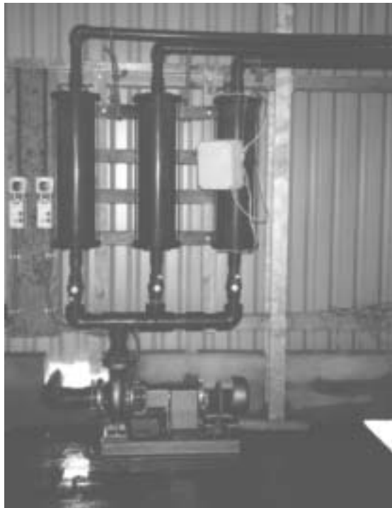
Pump and 3 x 6 lamp UV sterilizers
